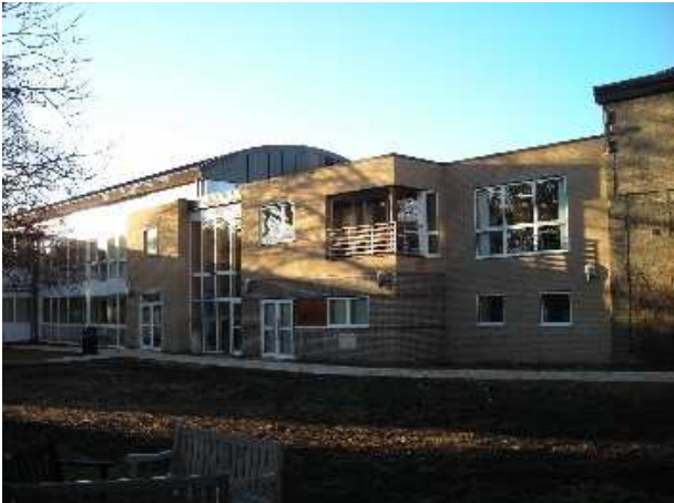
View from central garden area Images © Freeland Rees Roberts Architects.
