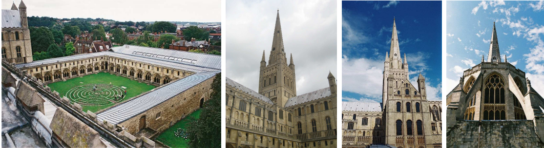
Major Conservation Work to Norwich Cathedral is Completed. Images by Freeland Rees Roberts Architects
